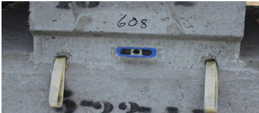
Slide Nut Embedded in Top of Panel
