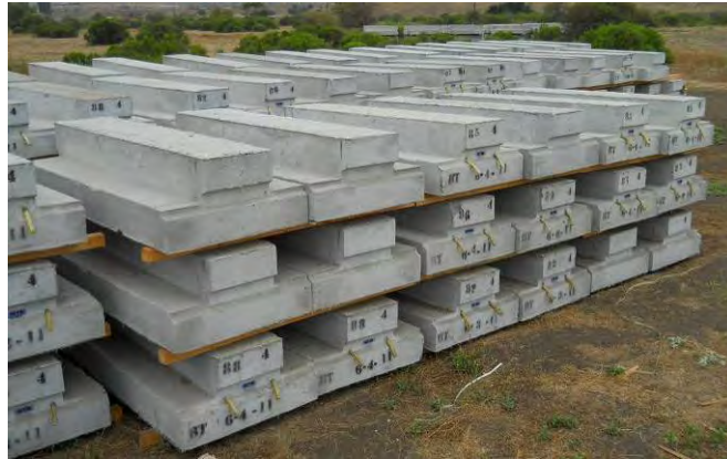
Stacked and Cribbed T Panels
