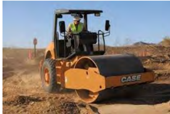
Compacting Earth Pad for SACON Structure
