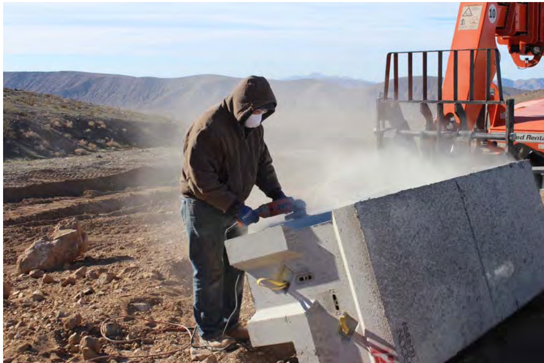
Grinding a Panel for Better Fit
