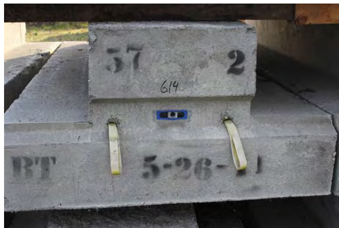
Lifting Straps on Finished T Panel
