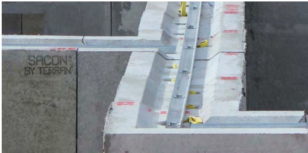
Picture of Steel Banding at Top of Keyed Panels
